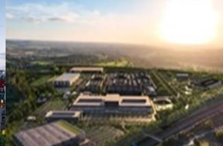
AiOnX data centre development fund
