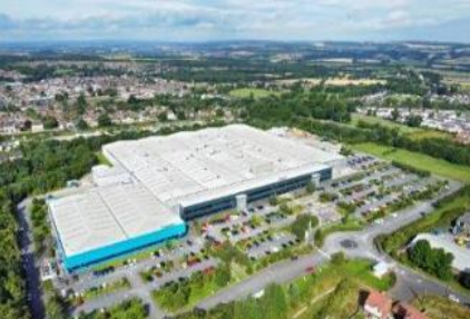
Thorn Lighting, Spennymoor, Durham, UK
